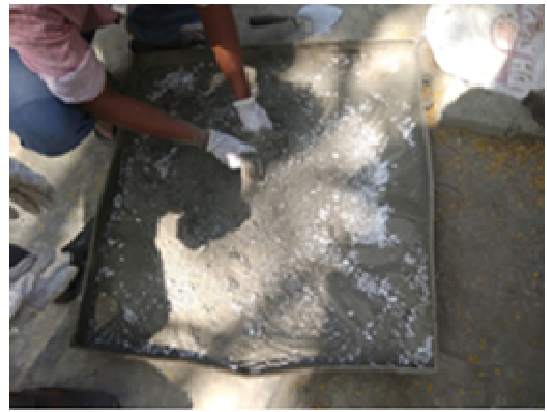
Fig 1. Dry mixing of concrete
