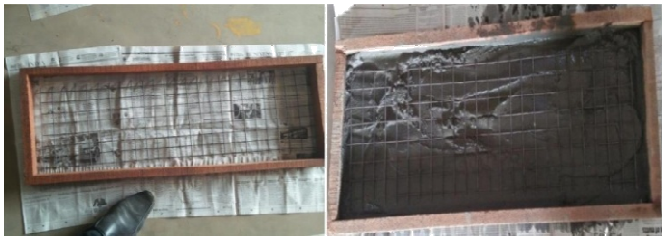
Fig. 1. Typical cross section of ferrocement structure
