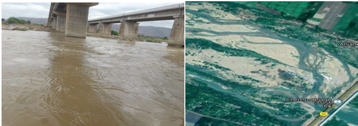
Site 2. Aadinimayapalle Dam across the Penna River in Chennur Village, YSR Kadapa district
